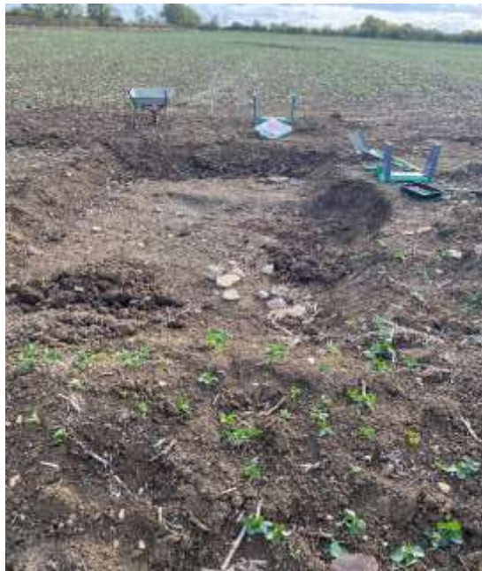
Trench 2 – Looking South
